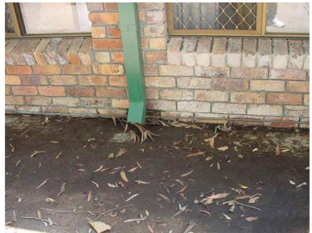
*Roof gutters not connected to approved stormwater outlets can cause damage to your property and neighbouring properties*
