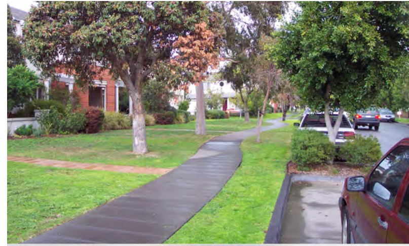
Figure 2 off-road trail incorporated into the road verge
