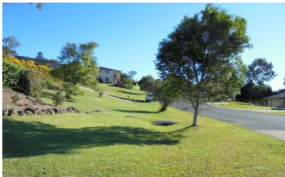
Figure 12 – Swale Drain Example: Perredenya Estate, Caniaba
