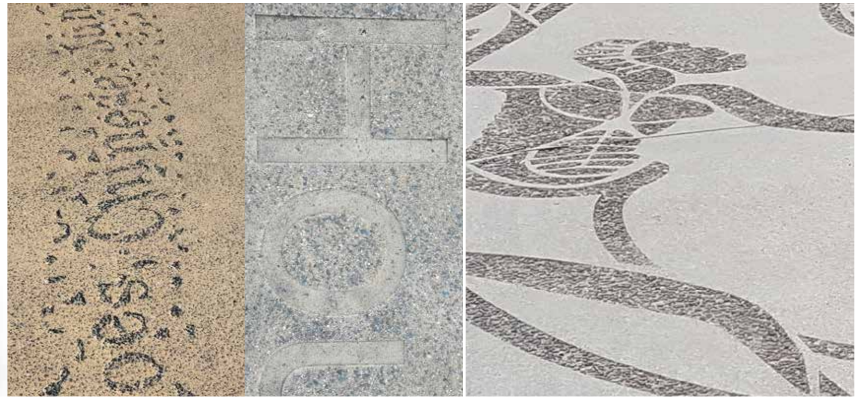
Character images; etched concrete. This process can be utilised for wayfinding and artworks and include coloured concrete and varying aggregate colours and textures
