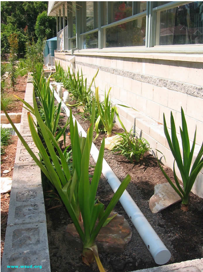
Plate 1.2 Bioretention planter box
