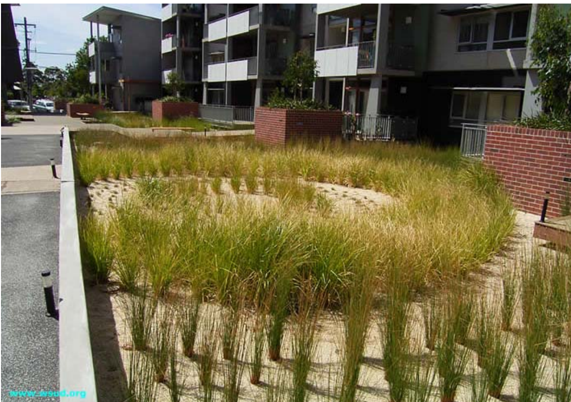
Plate 1.5 Bioretention basin in medium density development
