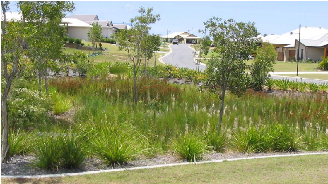
Plate 1.1 Bioretention basin in a streetscape setting
