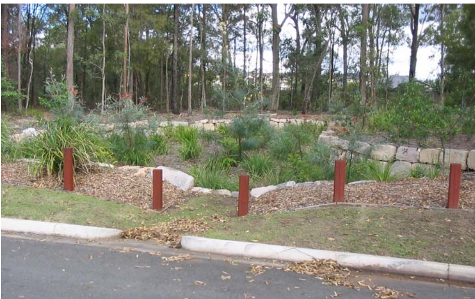
Plate 1.3 Bioretention basin with rock wall perimeter
