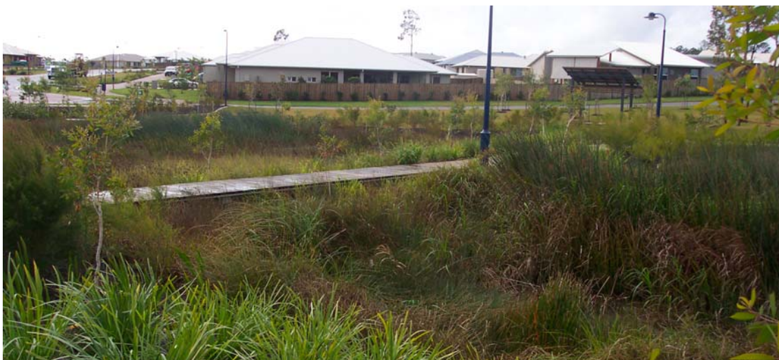
Plate 1.8 Constructed stormwater wetland with boardwalk
