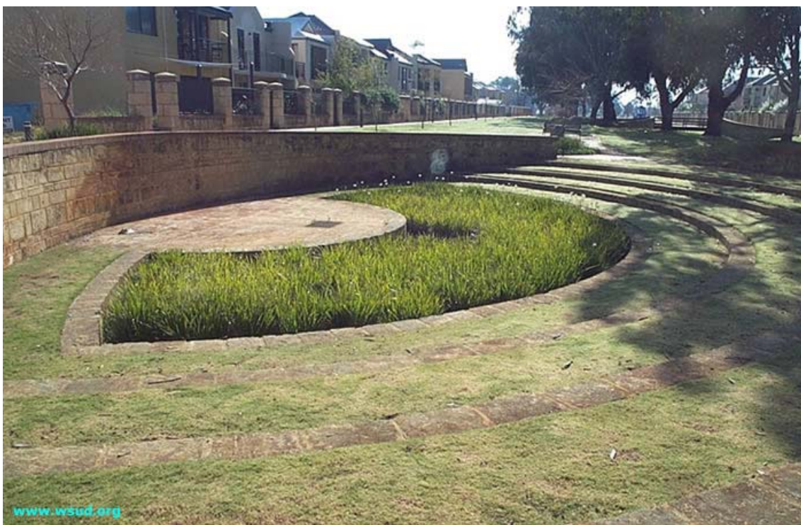
Plate 1.9 Constructed stormwater wetland in urban park setting
