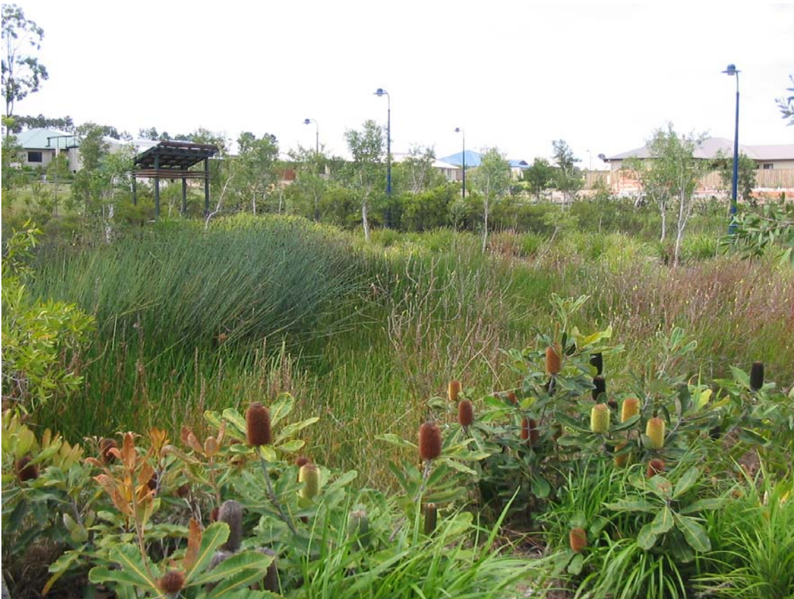
Plate 1.7 Constructed stormwater wetland in a residential setting
