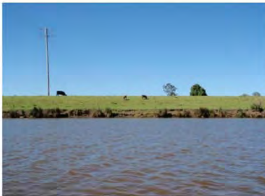
Plate 10: Bare riparian zone and active bank erosion along Tuckombil Canal
