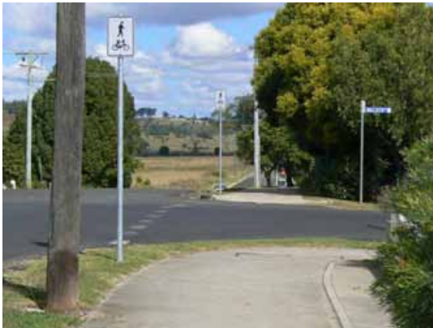
An existing off-road shared footpath along Walker Street in East Lismore
