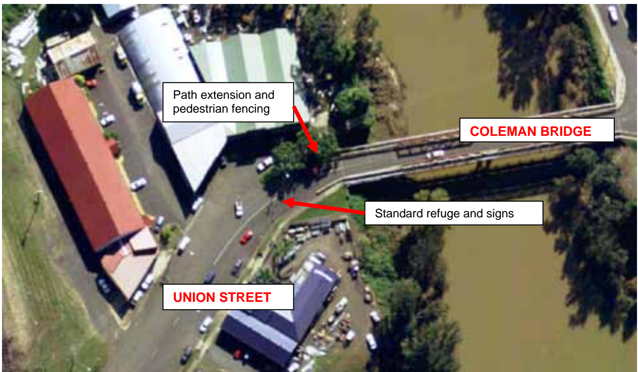
Item 9: Union Street approach to Coleman Bridge
