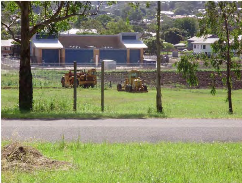
Plate 7: Westerly view towards Country Energy's substation.
