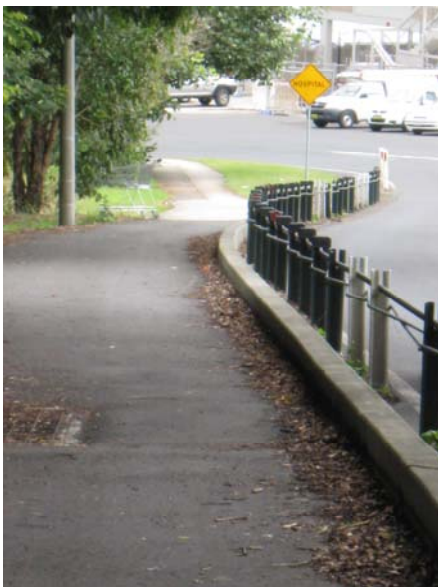
The Rotary Drive route constructed with Brifen safety fencing
