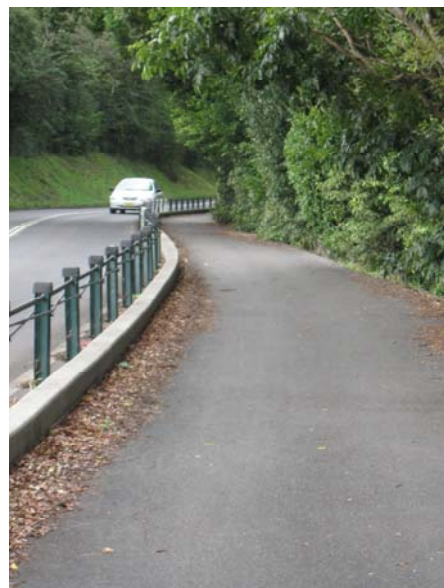
The Rotary Drive route constructed with Brifen safety fencing
