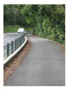
The Rotary Drive route constructed with Brifen safety fencing separating cyclists and pedestrians from the traffic lanes
