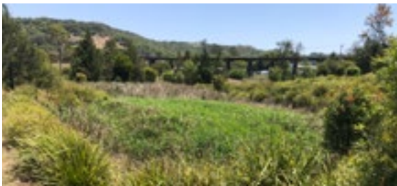
Constructed wetlands at Slaters Creek
