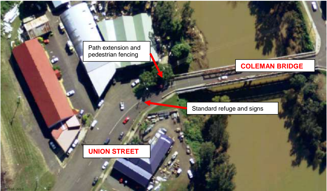
Item 12: Union Street approach to Coleman Bridge
