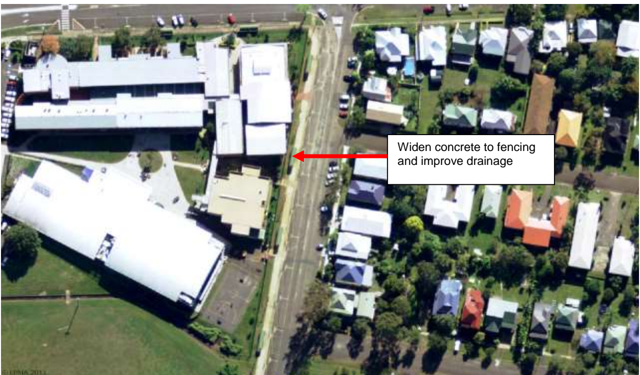
Item 56: Hindmarsh Street Bus Interchange
