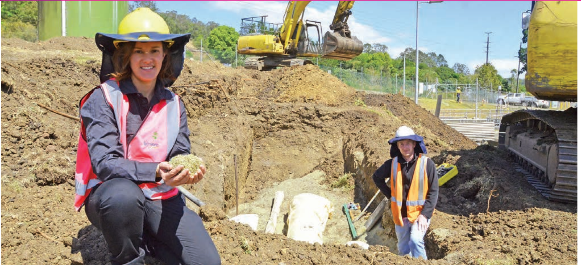
Use of recycled glass in construction.
