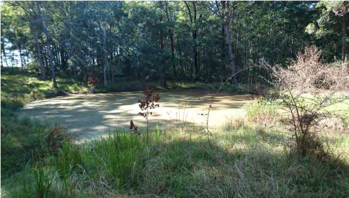
Dam on northern boundary of Zone e2 with evidence of maintenance by previous owner
