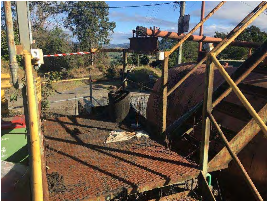
Figure 12. Remaining safety and access infrastructure after demolition of 27,000L diesel tank
