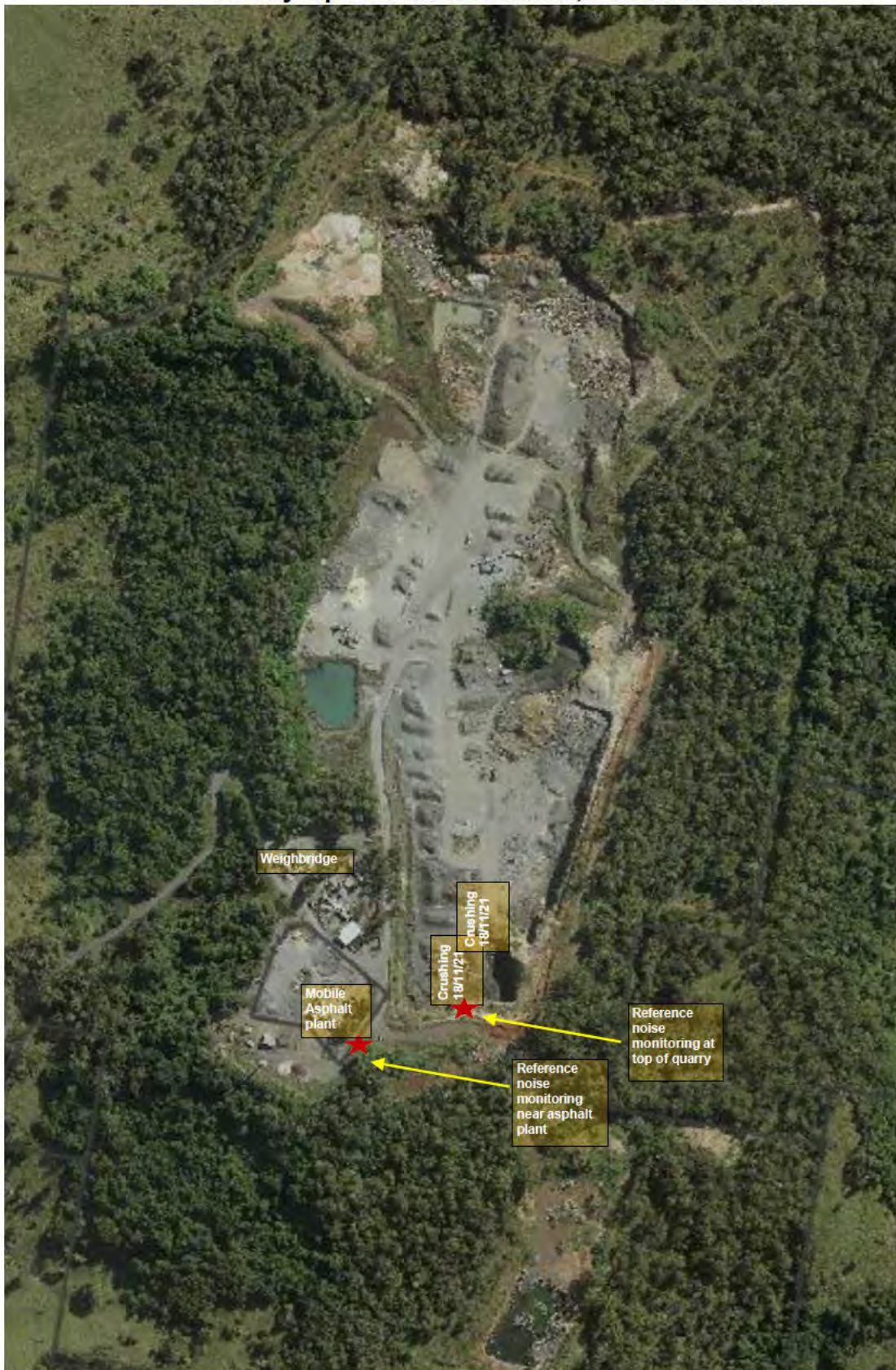
Image Source – Lismore City Council Online Mapping Note : Aerial photo not of November\, December 2021 operations
