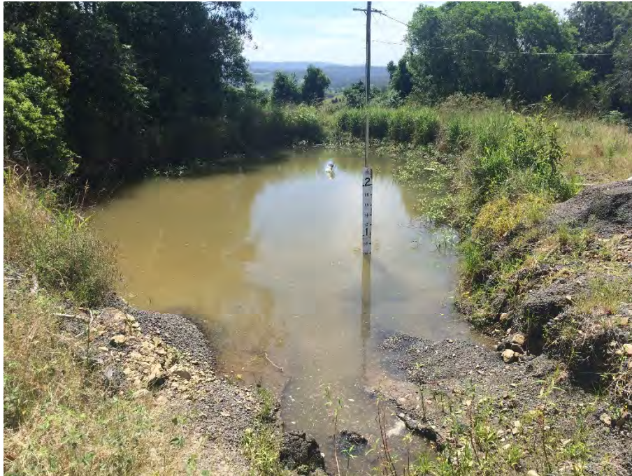
Plate 9: Sediment basin located near quarry entrance
