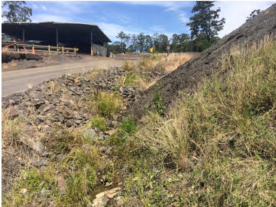
Plate 10: Drainage channel leading to sediment basin
