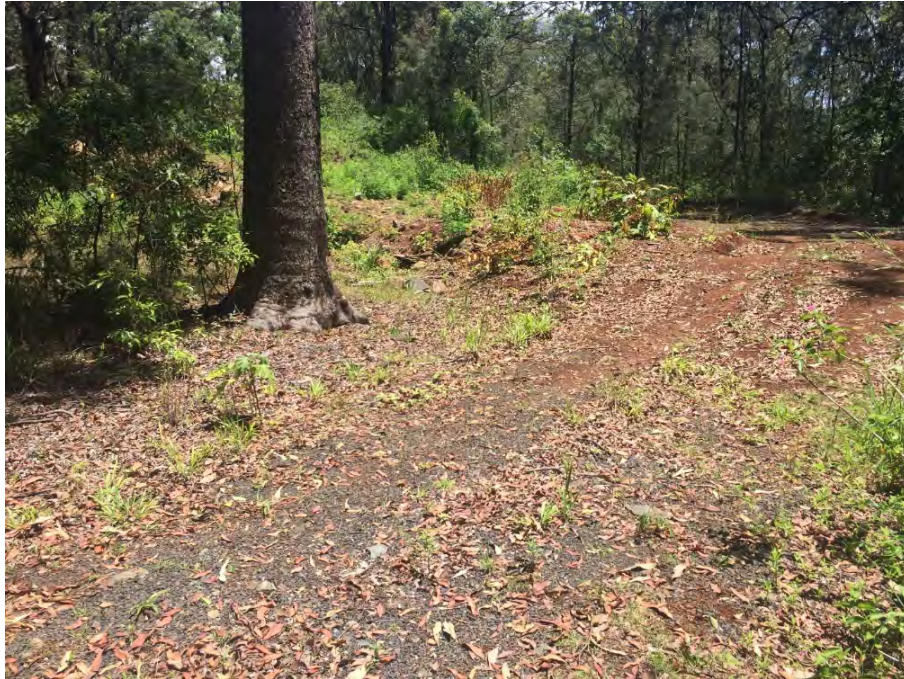
Plate 3: Upstream catchment diversion bund
