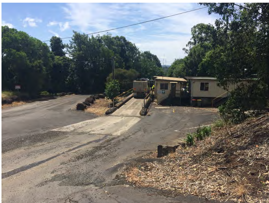
Plate 2: Weighbridge and offices
