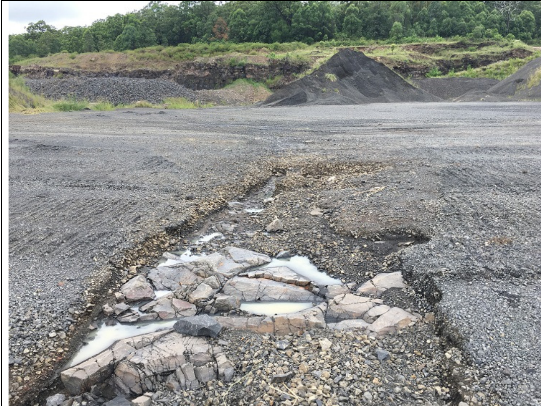
Plate 4 16/03/2017 Fractured basalt on Quarry floor near SW4.
