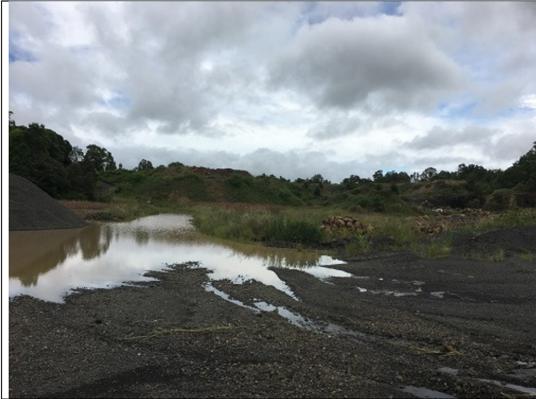
Plate 3 16/03/2017 Ponding of surface water near surface water discharge point SW4.
