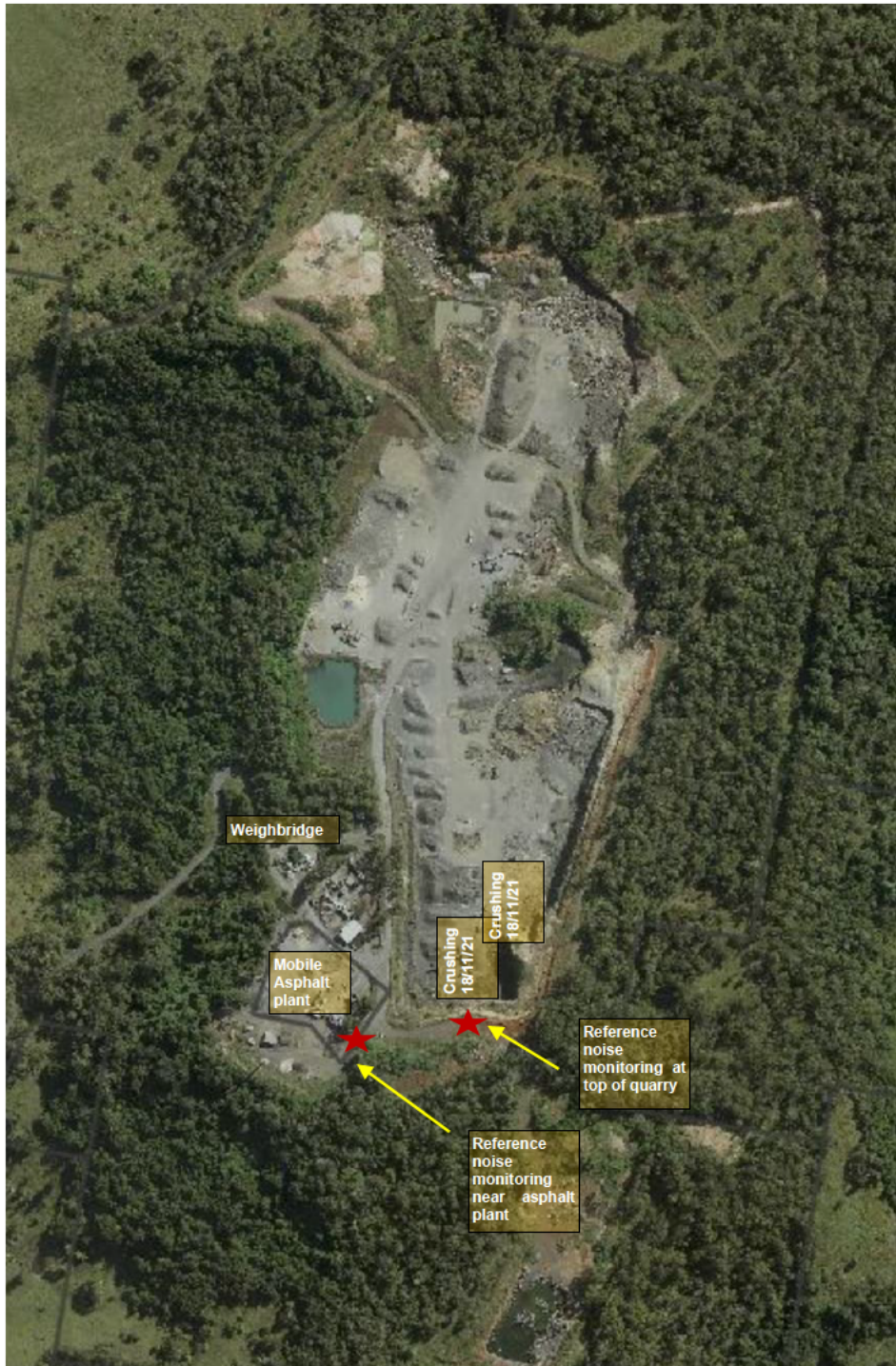
Image Source – Lismore City Council Online Mapping Note : Aerial photo not of November, December 2021 operations Quarry Pit Floor Operations 18 th November 2021
