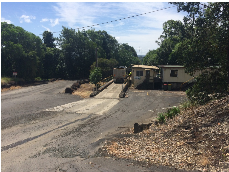
Plate 2: Weighbridge and offices
