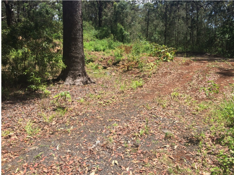
Plate 3: Upstream catchment diversion bund
