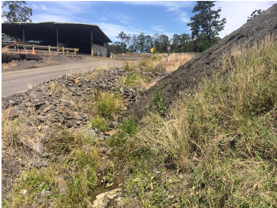
Plate 10: Drainage channel leading to sediment basin
