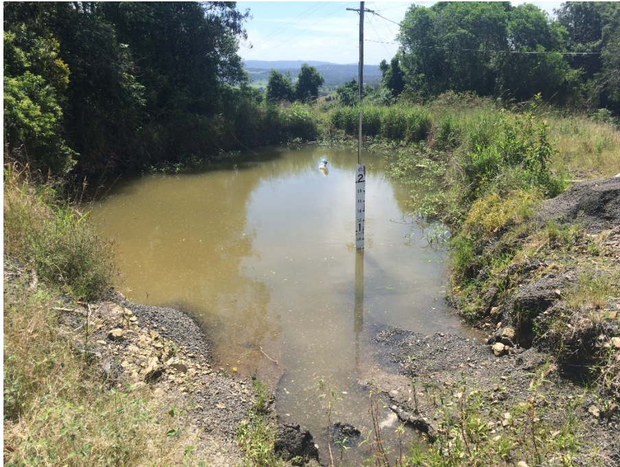
Plate 9: Sediment basin located near quarry entrance
