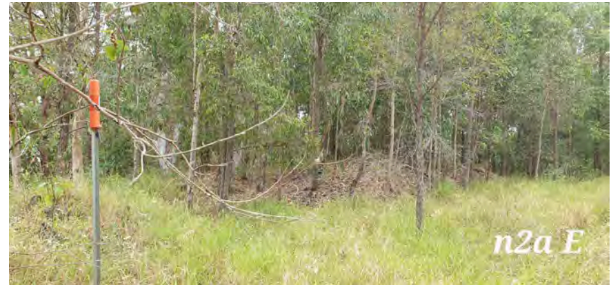
2022 East along northern boundary bund of zone n2
